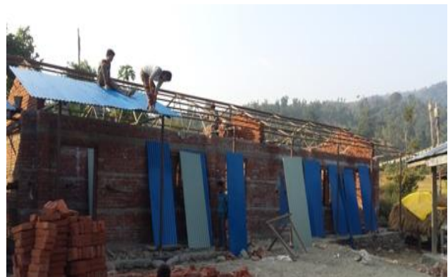
School Construction Work at Makwanpur District
