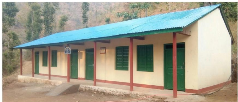
Newly constructed School Building of Saraswati P. School, Dokotar
