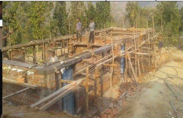
Kalidevi Primary School, Khairang-8 Tarling Building Construction
