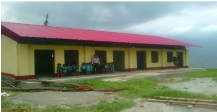
Newly built two room class room of Sarswati Primary School
